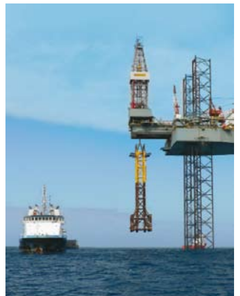
Installing the Kupe offshore platform
